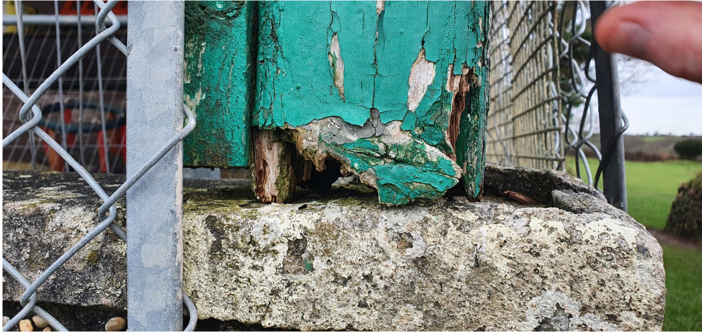
Roof support timber rotten and swaying in the wind could affect integrity.
