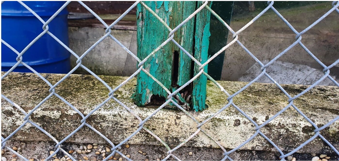
Another support timber rotten
