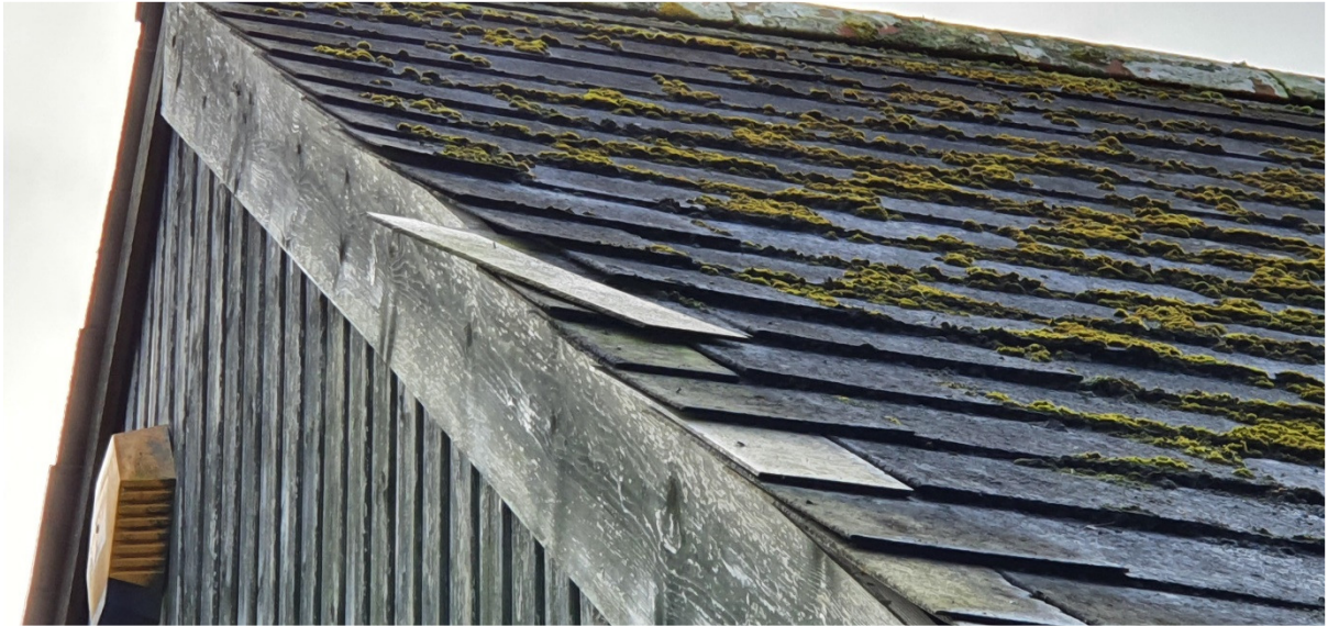
Loose roof tiles hazard in windy conditions and for the integrity of the building
