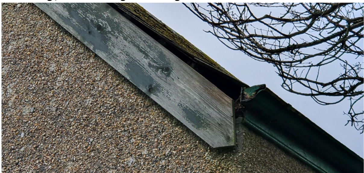
Fascia dropped, allowing birds to nest in the roof causing possible pressure on internal ceilings
