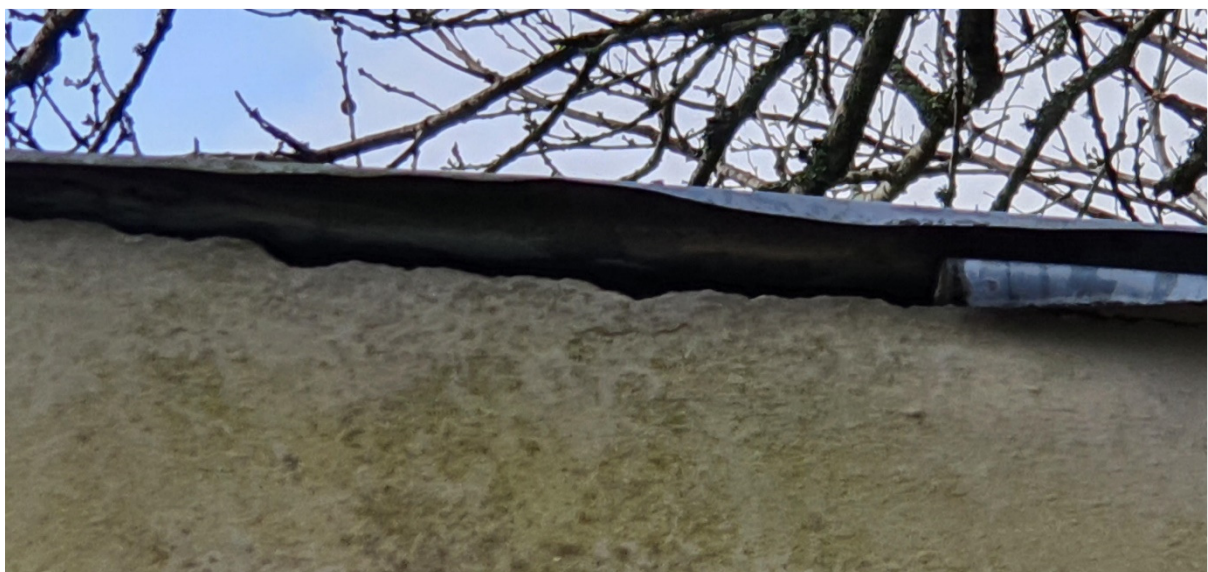
Roof lifted above rugby club shower block, could lift further in gales
