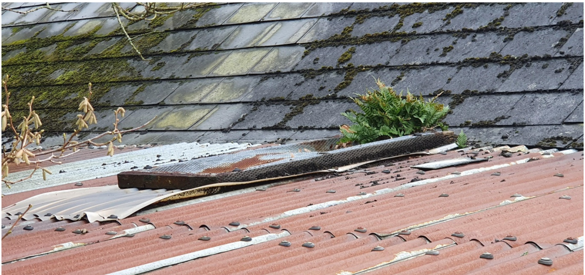
This picture shows a skylight which has holes in it, I believe someone stepping on it could fall through, it is on a low-level roof
