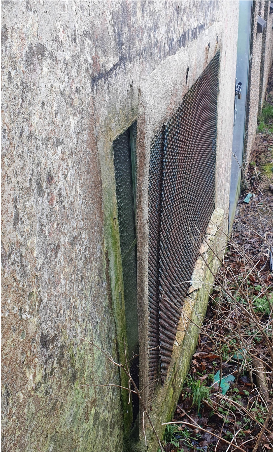
Protective metal grating coming away from wall
